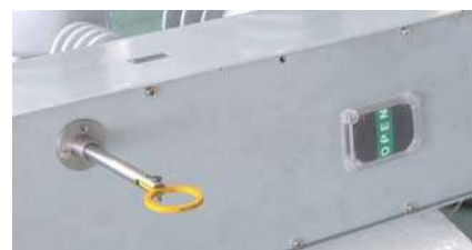
Lockout handle-pulled (open position)
