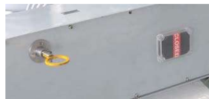
Lockout handle-push in (close position)
